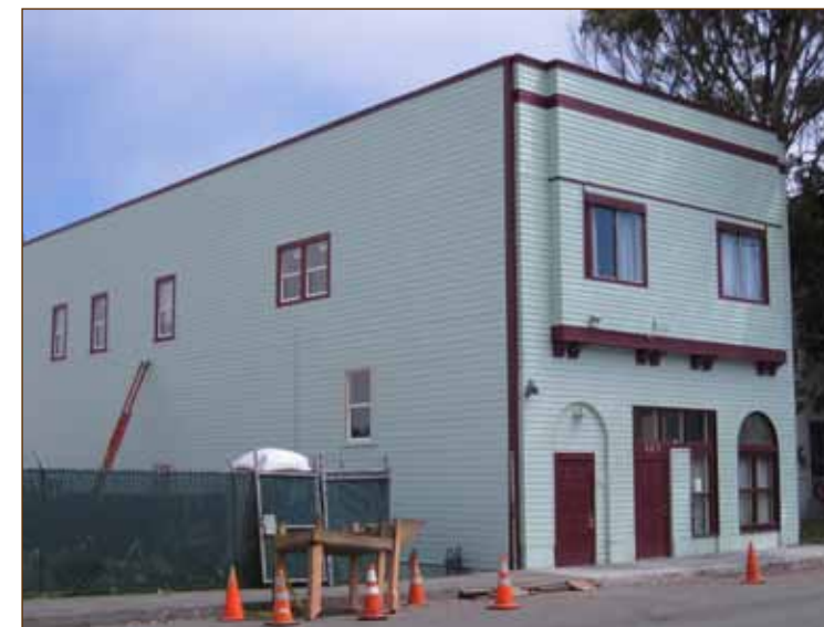
Siding installed, windows installed and painting completed as well
