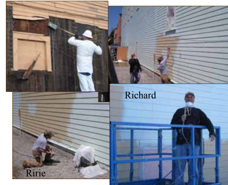
A work in progress, the many stages of the siding project
