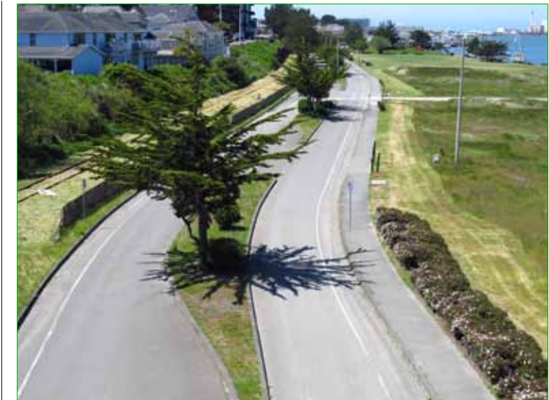
Completed weed abatement - behind library
